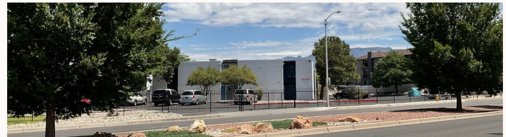
Before and after pictures of the Arioso Apartments. The property is now fenced and gated to limit access.
